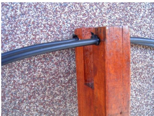
**Fig. 3.8** The loops are fixed with cable ties on both sides
